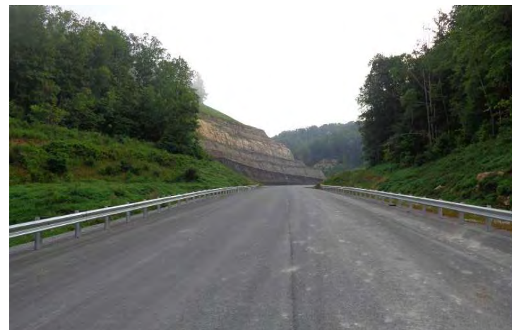
New US 460 Connector Roadway Base Asphalt & Temporary Guardrail
