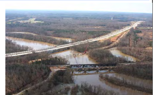
Construction of the new dual bridges over the Yadkin River.
