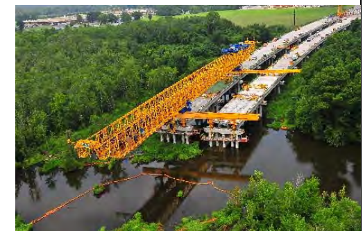
Custom-built gantries were used for top-down construction of the bridge.
