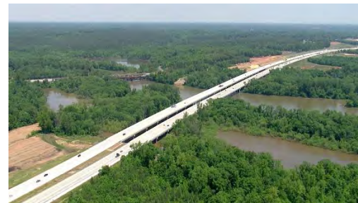
Completed new dual bridges over the Yadkin River.
