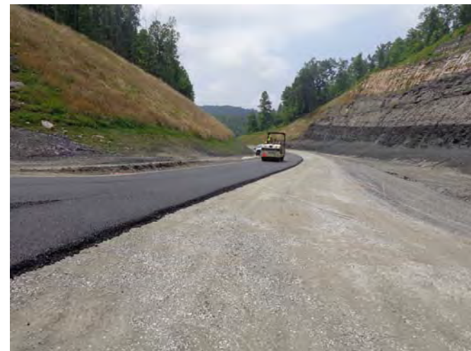
New US 460 Connector Roadway Pavement Placement
