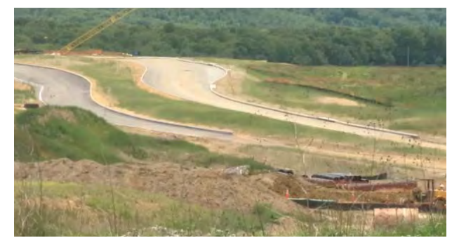
Relocated Southgate Drive (Route 314) under Construction
