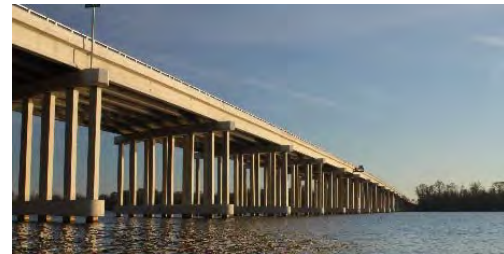
Completed 2.8-mile bridge over the Tar River.
