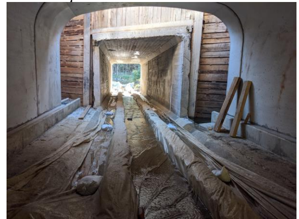
Figure 5.3: Rte 655 over Sulphur Spring Run Culvert Replacement
