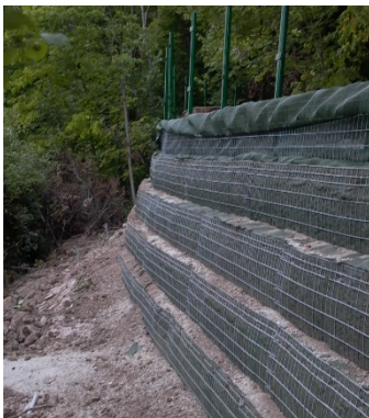
Figure 6 – Reinforced Slope Construction
