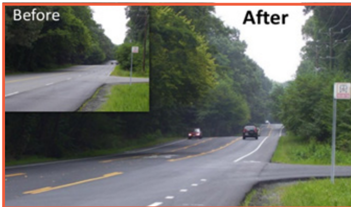
Lawyers Road Before and After.
