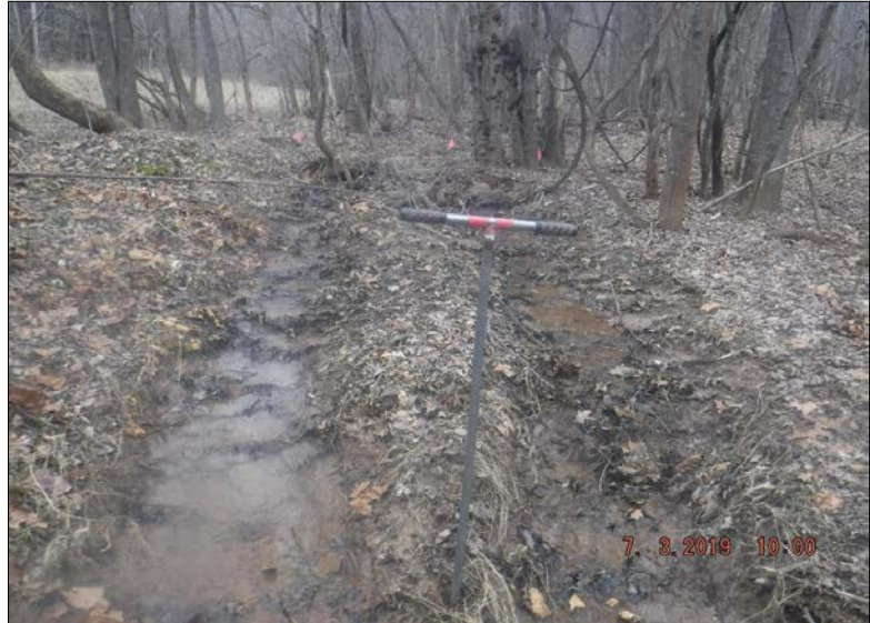
Looking southwest (upstream) at Stream Reach 76-A. The reach has some areas of erosion but the majority of the banks are stable. The right bank's riparian buffer has greater than 60% canopy cover with maintained herbaceous vegetation, while the left bank's riparian buffer is entirely forested with greater than 60% canopy cover. Stable habitat elements are present in 30-50% of the reach. The stream shows no signs of channel alteration.
