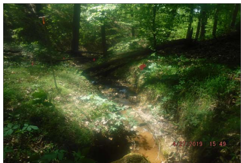
Looking downstream at Stream Reach 15-B. The stream is slightly incised and a majority of stable banks with 60-80% vegetative surface protection. The left and right bank riparian buffers consist of mature forest with greater than 60% tree canopy cover. Instream habitat is present in less than 10% of the stream. No channel alteration is present within the stream.
