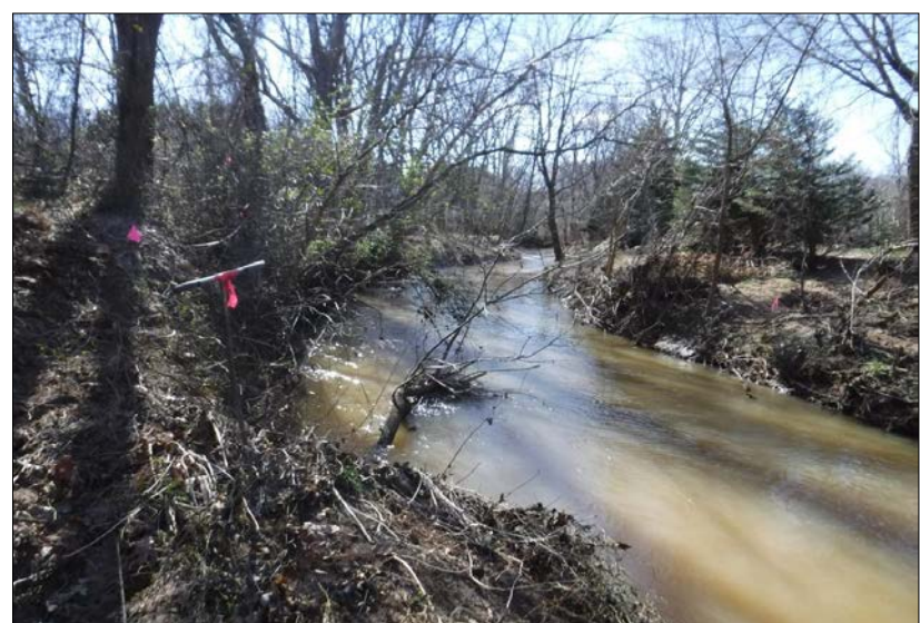
Looking upstream at Reach 10-A (Marrowbone Creek). The reach was suboptimal with stable and vegetated banks and a few areas with active erosion. The right riparian buffer consisted of 30% mature forest with wetlands and 70% non-maintained herbaceous areas. The left riparian buffer consisted of 95% maintained residential lawns and 5% impervious surface associated with parking lots and roads. The in-stream habitat consisted of riffles, pools, leaf packs and various particle sizes, however, the stream was degraded by aggregation and pollution. The reach was riprapped and channelized through culverts.
