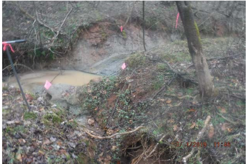
Looking downstream at Stream Reach 138-A. The reach was severely incised with active erosion throughout. The right and left riparian buffer consisted of 100% optimal canopy cover. The instream habitat was poor throughout the reach, lacking riffles, pools and leaf packs. The reach had no channel alterations.
