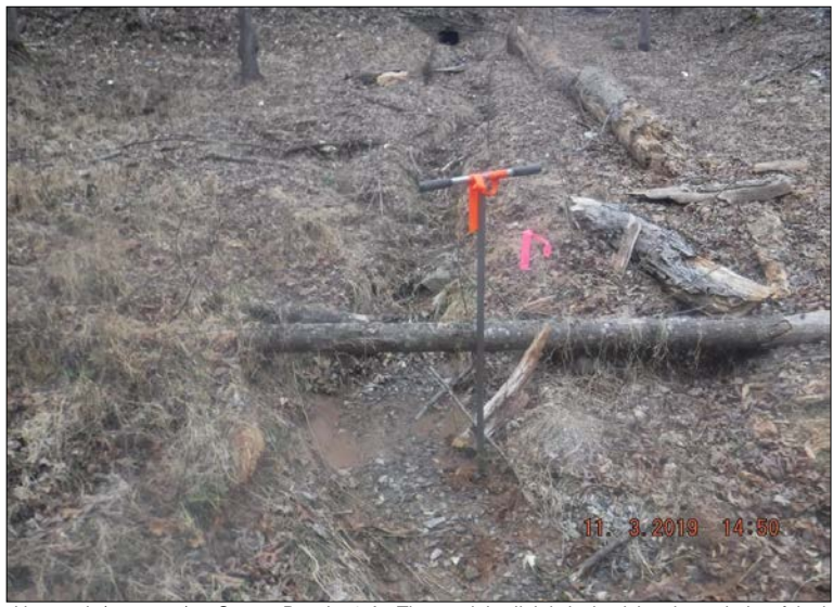
Looking north (upstream) at Stream Reach 59-A. The reach is slightly incised, but the majority of the banks are stable (60-80%). The right and left riparian buffers are composed of tree canopy cover between 30-60% and a non-maintained understory. Stable habitat elements are present in 10-30% of the reach. The upstream end of the reach is fed by a culvert, disrupting less than 20% of the reach.
