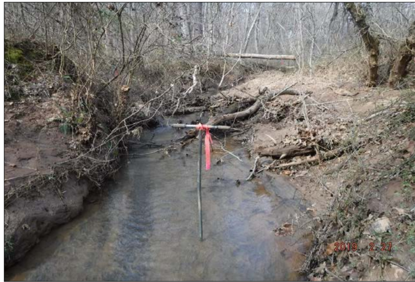
Looking upstream at stream reach 88-A. The reach was slightly incised with majority of banks stable. The right riparian buffer consisted of 98% mature forest cover and 2% herbaceous field. The left riparian buffer contained 88% mature forest cover, 2% non-maintained dense vegetation, and 10% herbaceous field. The in-stream habitat was suboptimal with stable elements in 30-50% of the reach, and the channel had no alterations.
