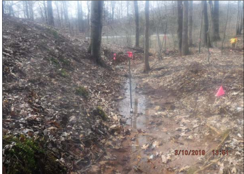
Looking southwest (downstream) at Stream Reach 63-A. The banks are slightly incised with mostly stable banks (60-80%). The right bank's riparian buffer is predominantly forested, with an area of dense herbaceous vegetation and shrubs providing less than 30% tree canopy cover. The left bank's riparian buffer is composed of forest with greater than 60% tree canopy cover. Instream habitat elements are stable and present in 30-50% of the reach. The downstream end of the reach is culverted, disrupting 20-40% of the reach.
