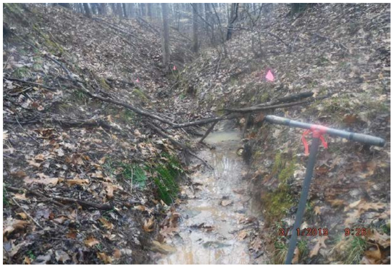
Looking upstream at Stream Reach 133-B. The reach was moderately incised with areas of active erosion. The right and left riparian buffer consisted of 100% optimal canopy cover. The instream habitat consisted of riffles, pools, leaf packs and substrate of various particle size but had excess sediment and silt due to active erosion. The reach had no channel alterations.
