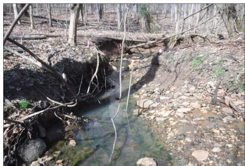
Looking upstream at Stream Reach 6-A. The reach was incised with active erosion at the culvert at the top of the reach. The riparian buffers consisted of 80% mature tree cover and 20% impervious surfaces associated with State Route 220. Instream habitat is present in 10-30% of the reach and consisted of riffles, pools, leaf packs and substrate of various particle sizes. The channel was riprapped at the culvert.
