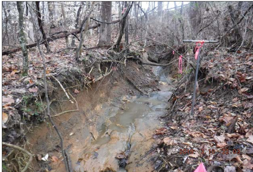
Looking upstream at Reach 19-B. The reach channel was rated severe with frequent areas of active erosion and acute aggregation. The riparian buffers consist of 10% maintained lawns and 90% mature forested areas. In-stream habitat was present in less than 10% of the reach. The reach was channelized through culvert and riprapped for stability at the top of the reach.
