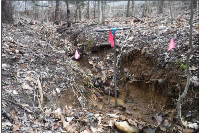
Looking upstream at stream reach 34-A. The reach was poor frequent areas of active erosion. The riparian buffers consisted of 75% mature forested cover and 25% impervious surfaces associated with State Route 220. Instream habitat was degraded by erosion and is present in less than 10% of the reach. The reach was channelized through culverts.
