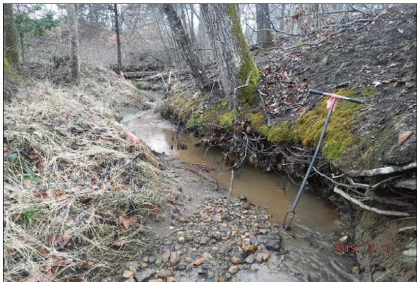
Looking downstream at stream reach 106-A. The reach was incised with some erosion and vegetative protection present. The right riparian buffer consisted of 25% mature forest cover, 5% maintained vegetation, and 70% denuded clear cut land. The left riparian buffer contained 20% mature forest cover, 10% maintained vegetation, and 70% denuded clear cut land. The in-stream habitat was marginal with stable elements in 10-30% of the reach, including cobbles, undercut banks and shade. No channel alterations were observed.
