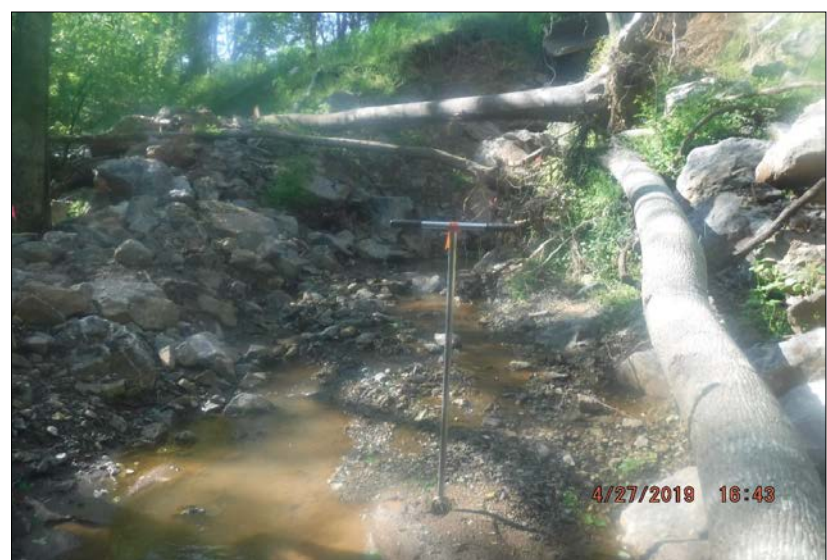
Looking upstream at Stream Reach 1-B. The stream is often incised with erosion present on both banks. The left bank riparian buffer consists of mature forest with greater than 60% tree canopy cover and impervious surfaces. The right bank consists of a wetland and mature forest with greater than 60% tree canopy cover. Instream habitat is present in less than 10% of the stream. Channel alteration is present in 60-80% of the reach from a concreted culvert and rip-rap.
