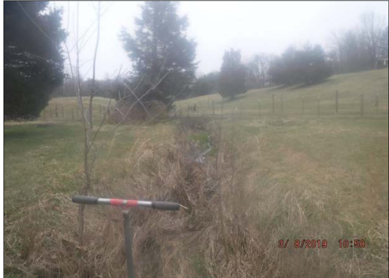
Looking south (downstream) at Stream Reach 64-D. Both banks' riparian buffers consist of actively grazed pasture. Instream habitat elements are lacking, and are present in less than 10% of the reach. The upstream end of the reach is fed by a culvert, disrupting less than 20% of the reach.
