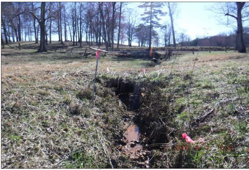
Looking upstream at stream reach 52-B. The reach had severely eroded, unstable banks. The right riparian buffer consisted of 55% maintained pasture, 15% impervious surface and 30% wetland. The left riparian buffer consisted of 90% maintained pasture and 10% wetland. The in-stream habitat was poor and lacked stable elements. Channel alterations were severe and included multiple culverts, straightening of channel and impacts from livestock.
