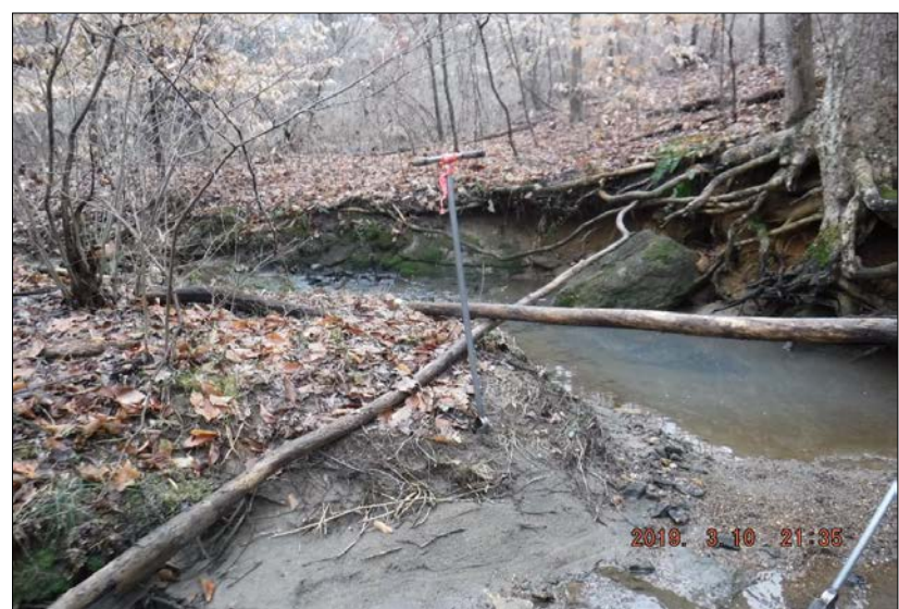
Looking upstream at stream reach 23-A. The reach was incised with active erosion throughout. The right riparian buffer consisted of 100% mature tree cover. The left riparian buffer consisted of 100% mature tree cover. Instream habitat was present in 30-50% of the reach. The reach was channelized through culvert at the top of the reach.
