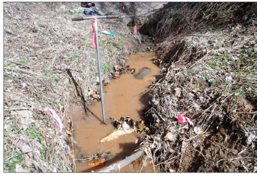
Looking upstream at stream reach 113-C. The reach had incised and eroded banks. The right riparian buffer consisted of 40% mature forested cover and 60% maintained vegetation. The left buffer contained 98% maintained vegetation with kudzu cover and 2% PEM wetland cover. The in-stream habitat was poor, containing leaves and few pools. No channel alterations were observed.
