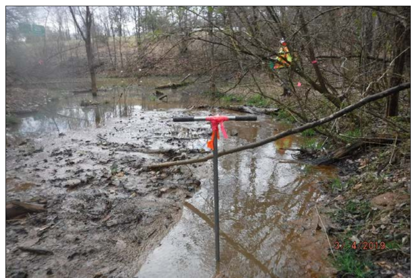
Looking downstream at Stream Reach 4-A. The reach was level with stable banks and had few areas of active erosion, however severe aggregation was present due to restricted flow at the culvert crossing near State Route 220. The riparian buffers consisted of 50% mature tree cover with wetlands and 50% impervious surface associated with State Route 220. The in-stream habitat is present in less than 10% of the reach. Channel alteration was present at a riprapped culvert.
