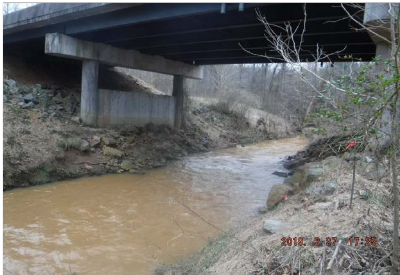
Looking upstream at stream reach 91-A. The reach had eroded banks and was overwidened, with little vegetative protection present. The right and left riparian buffers consisted of 60% mature forest cover and 40% impervious surfaces associated with Soapstone Road. The in-stream habitat was suboptimal with stable elements in 30-50% of the reach, and channel alterations included road and brige installation.
