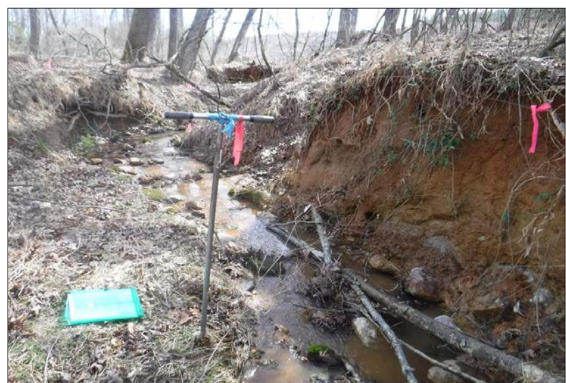
Looking downstream at stream reach 40-A. The reach was poor with frequent areas of active erosion. The riparian buffers consisted of 25% mature forested areas and 75% impervious surfaces associated with State Route 220. Instream habitat was present in less than 10% of the reach and consisted of riffles, pools, leaf packs, and head-cuts, however, the reach was degraded by severe aggregation and active erosion. The reach was channelized through a culvert.
