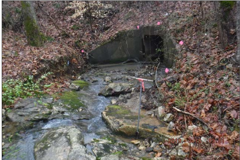
Looking downstream at 20-B. The reach was suboptimal with minor area of active erosion throughout with stable and vegetated banks. The right riparian buffer consisted of 100% mature tree cover. The left riparian buffer consisted of 70% mature tree cover and 30% densely non-maintained herbaceous area. Instream habitat was present in 30-50% of the reach and consisted of riffles, pools, head cuts, leaf packs and substrate of various particle sizes. The was channelized through culverts at the top and bottom of reach.
