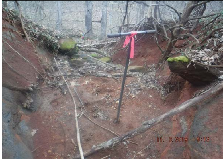
Looking east (downstream) at Stream Reach 66-A. The channel is deeply incised, restricting flow to within the banks. Both riparian buffers are composed of forest providing greater than 60% tree canopy cover. Habitat elements are unstable and are present in less than 10% of the reach. A culvert is disrupting less than 20% of the reach.
