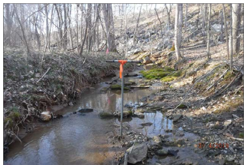
Looking upstream at Stream Reach 1-A. The reach was incised with active erosion at a culvert. The right riparian buffer consisted of 80% mature tree cover and 20% impervious surfaces associated with State Route 220. The left riparian buffer consisted of 100% mature tree cover. The instream habitat was present in 30%-50% of the reach and consisted of riffles, pools, leaf packs and substrate of various particle sizes. The channel was riprapped at the culvert upstream.
