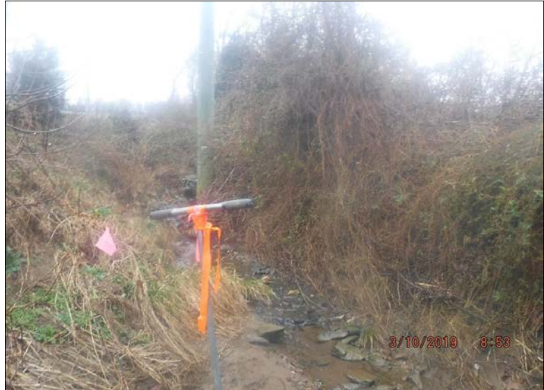
Looking north (upstream) at Stream Reach 72-A. Active erosion is occurring, with vegetative protection on 40-60% of the banks within the reach. Both riparian buffers are encroached upon by paved asphalt, with dense herbaceous vegetation occupying the space between the stream and pavement. Stable habitat elements are present in 10-30% of the reach. The reach is culverted across Joseph Martin Highway (Rt. 641) and the upstream end of the reach is fed by a culvert, disrupting 20-40% of the reach.
