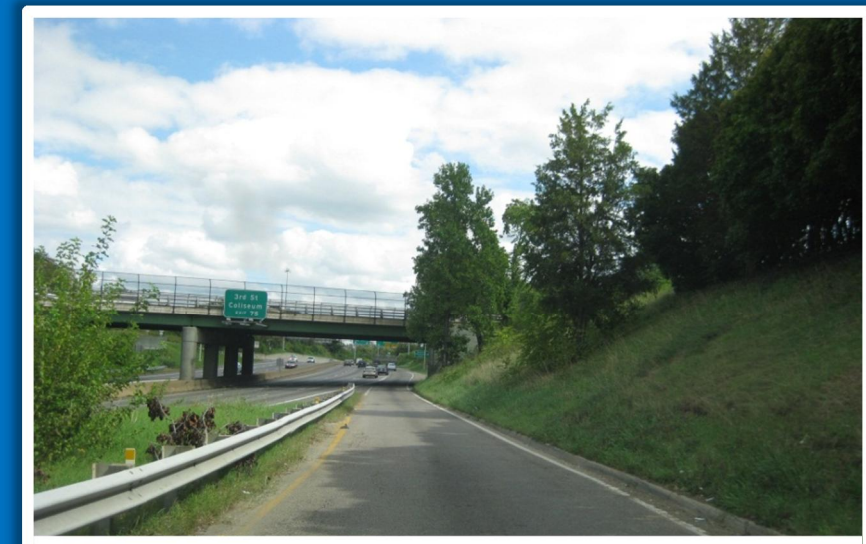
Photograph 3 – Looking East from Merge Point of Upstream On-Ramps from Belvidere Street
