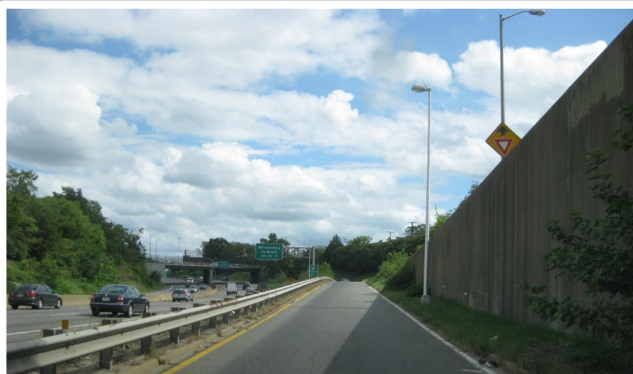
Photograph 1 – Looking East from CD Road from Belvidere Loop On-Ramp
