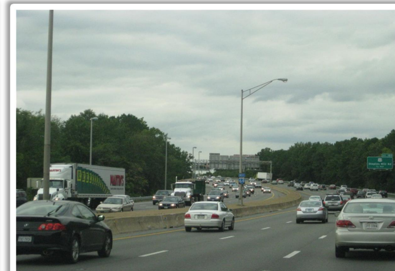
Photograph 2: I-64 West of Bryan Park Interchange – Conventional Roadway Lighting
